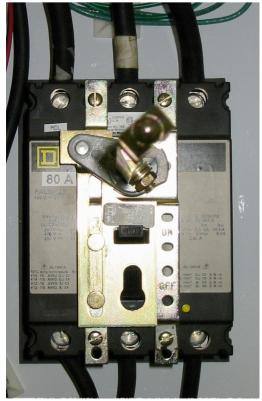
480 VAC 80 Amp service should be connected to the top of the main breaker and ground line to Main ground lug.
